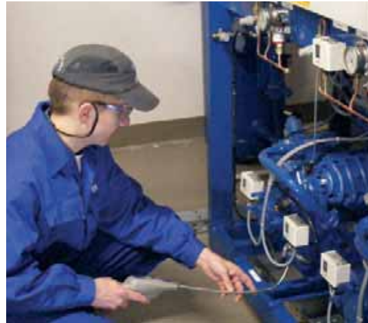
Leak test by service engineer with electronic leak detector
